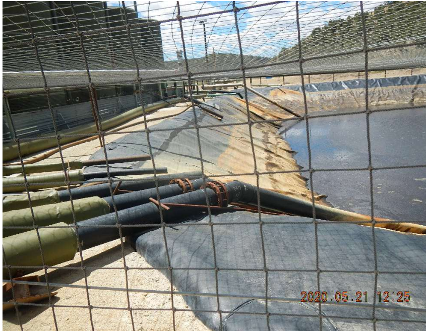
Hoses, pipes, and metal directly on pit liner.
