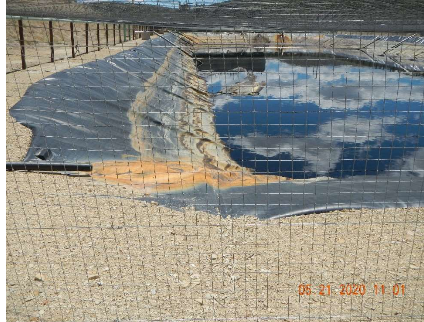
Sediment encroaching on pit liner and poly line directly on pit liner
