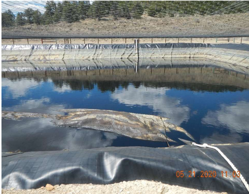
Pit liner bubbling up to the fluid level surface
