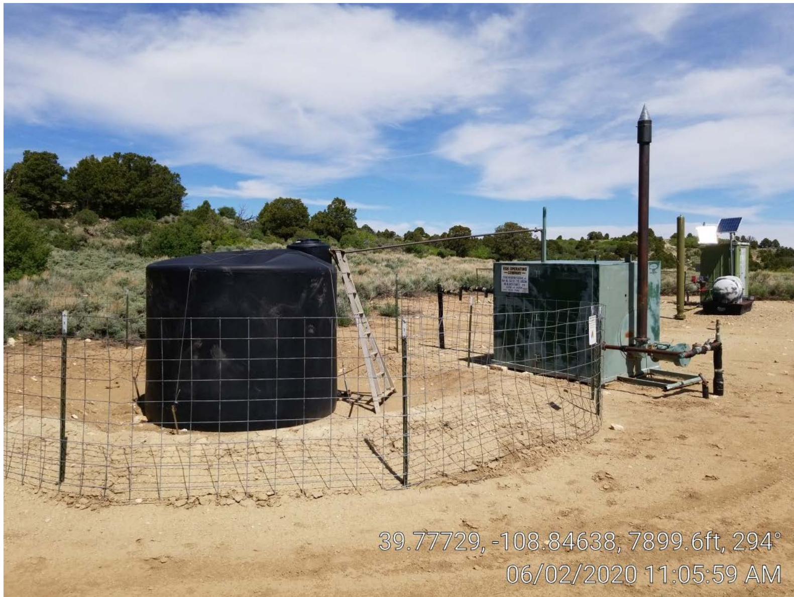
Photo 2. Tank, separator, and meter building.
