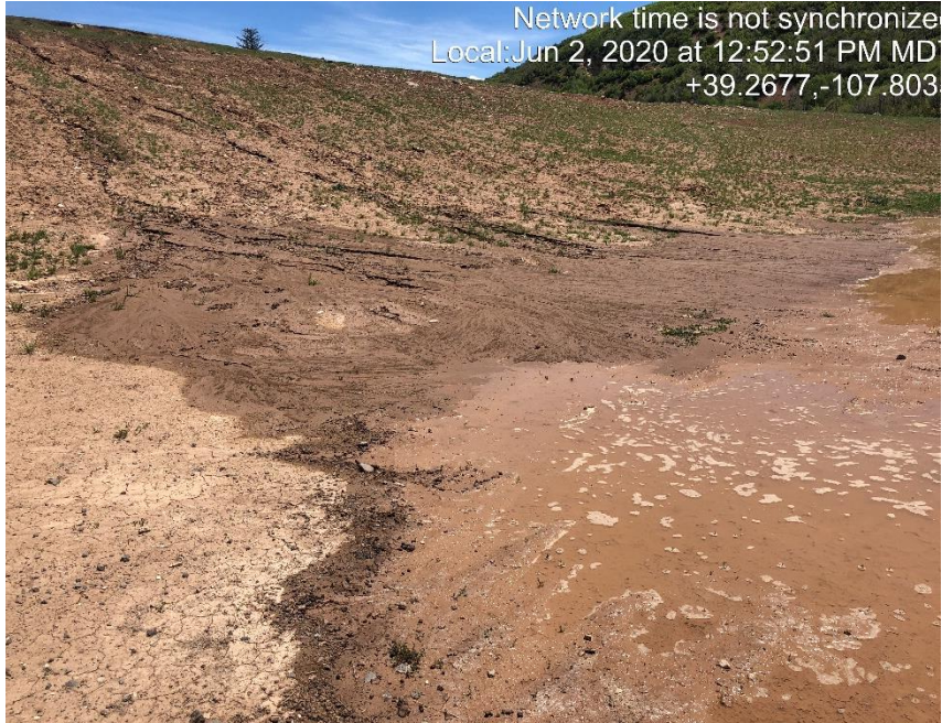
Photo #1295 Sediment moving on to location from South West cut slope.
