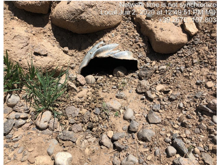
Photo #1294 Sediment build up in culvert at entrance to location.
