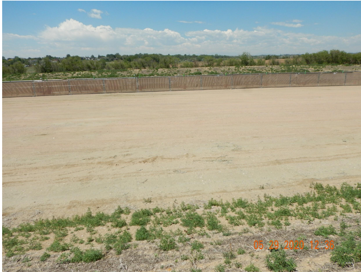
Photo 8. Photo taken from the western set of wells, facing West. Photo illustrates Operator has performed interim reclamation activities to reduce disturbance areas only needed for production operations.
