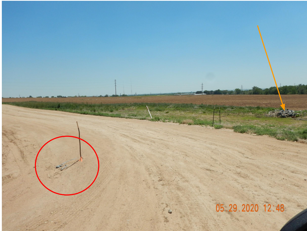
Photo 11. Photo taken from the southern location, facing Southeast. Photo illustrates a culvert needing repair. Culvert directs stormwater to a stabilized outlet area (orange arrow).
