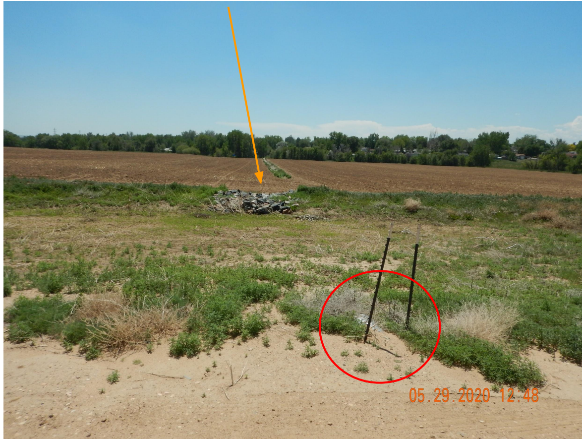
Photo 12. Photo taken from the southern location, facing South. Photo illustrates the outlet of the culvert that directs stormwater to a stabilized outlet area (orange arrow).
