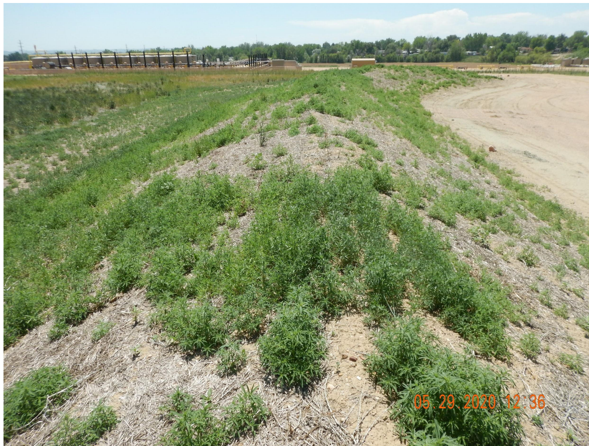
Photo 9. Photo taken from the western set of wells, facing South. Photo illustrates a stockpile that has been temporarily stabilized with equipment tracking. Operator has attempted to seed into the stockpile with the evidence of drill rows and straw crimped mulch. However, there was little establishment of desirable species and currently has mostly Kochia establishment.
