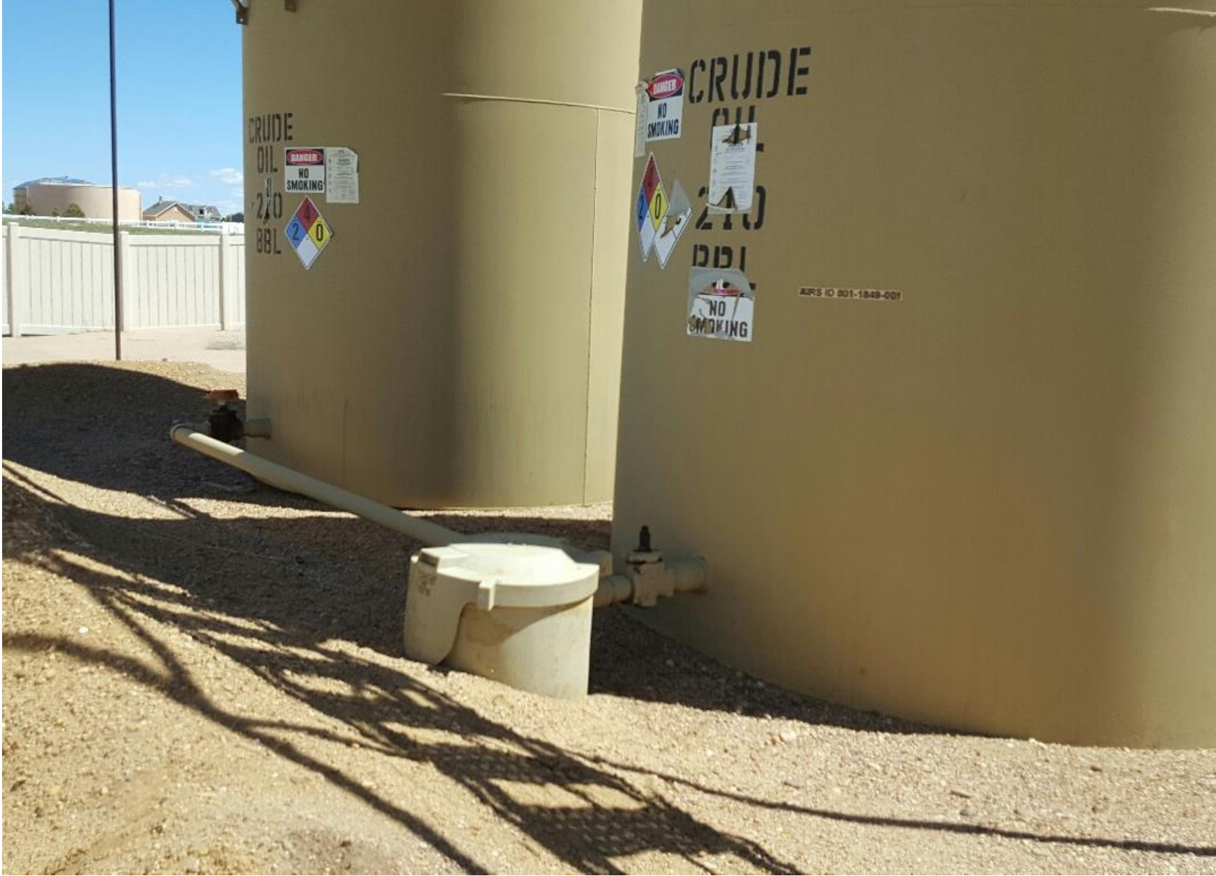
Figure #2 Bull plug has been installed.
