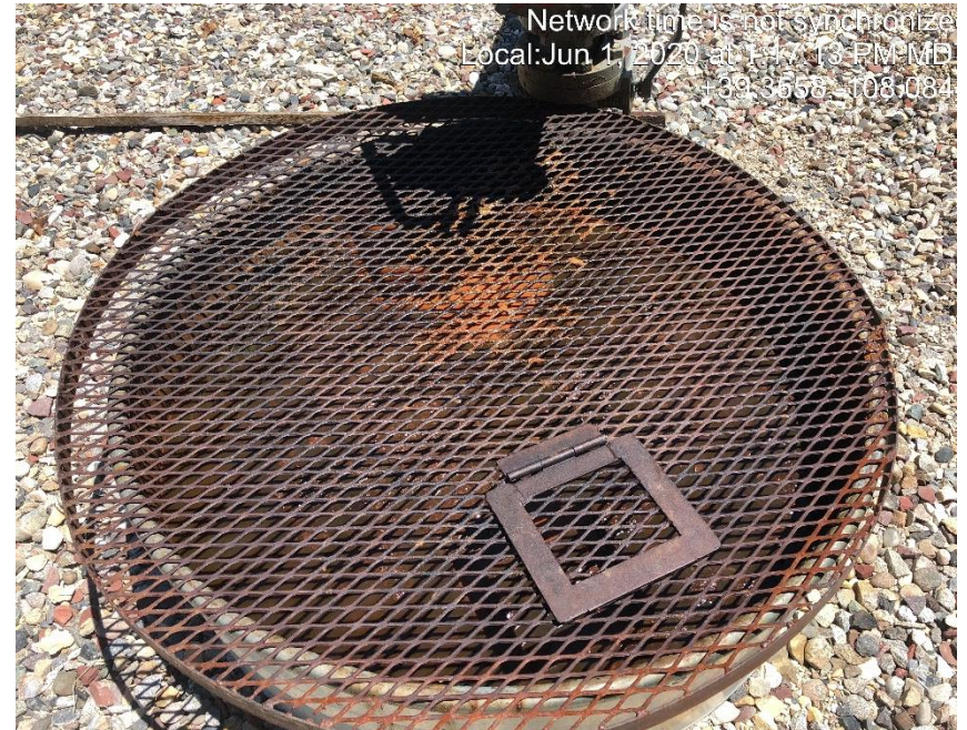
Photo #1286 Oily fluid in containment by pigging station.
