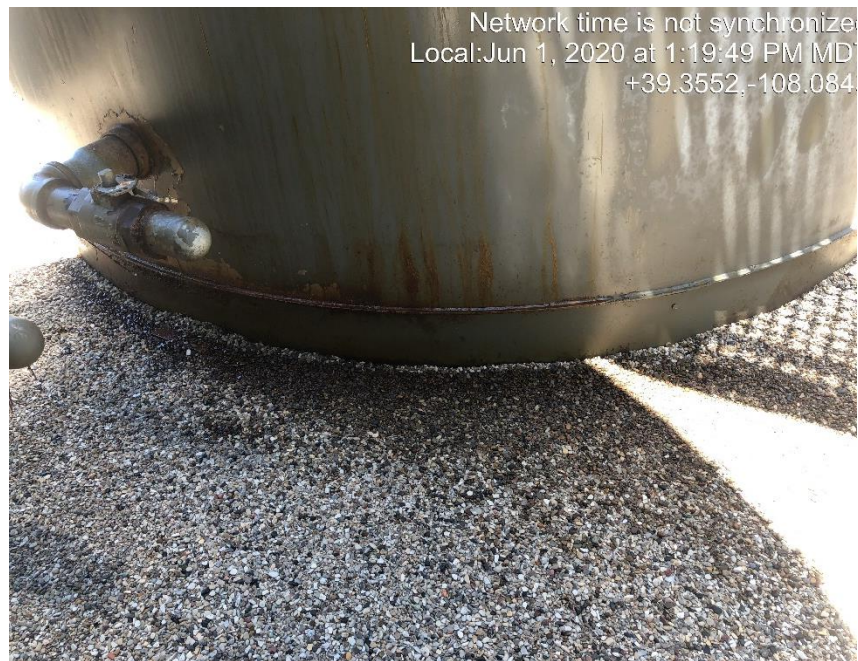
Photo #1287 stained gravel in tank containment.
