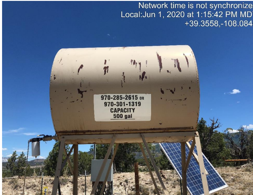
Photo #1284 500 gallon methanol tank missing operators name.
