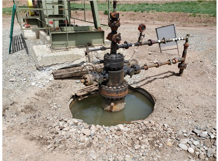
Photo 12: Photo of the 051-06129. Photo shows containment has filled with fluid and requires maintenance.
