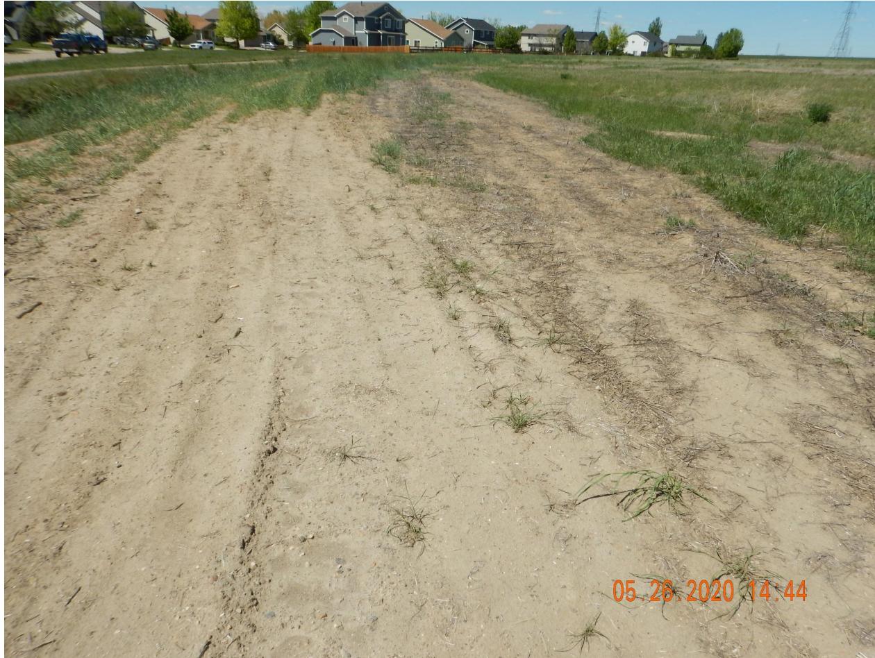
Photo 1. Photo taken from the southern access road, facing North. Photo illustrates the Operator attempted to conduct final reclamation activities; however, little to no establishment of desirable plant species was observed throughout much of the access road and well location.
