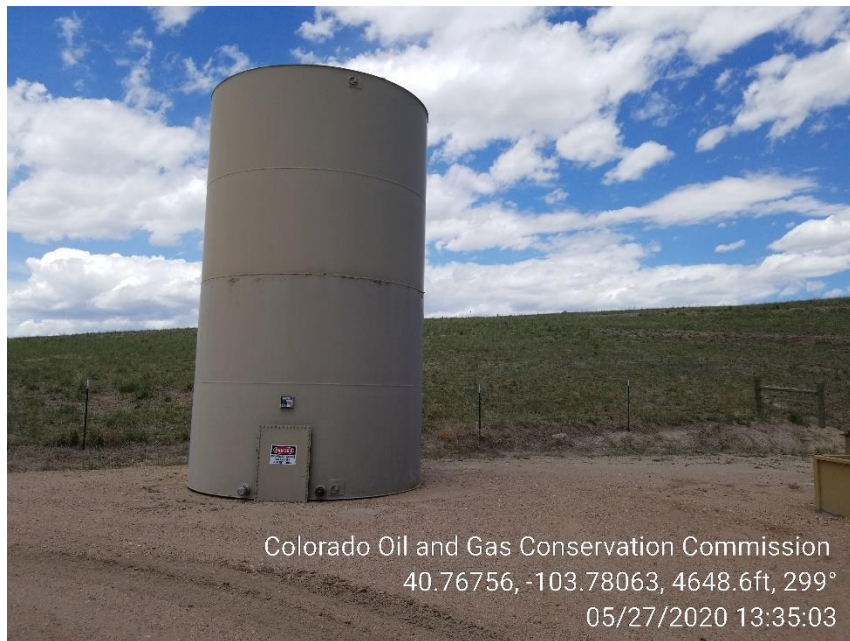
Photo 3 – Unused 400 BBLS Crude Oil Tank on the Northside of Location
