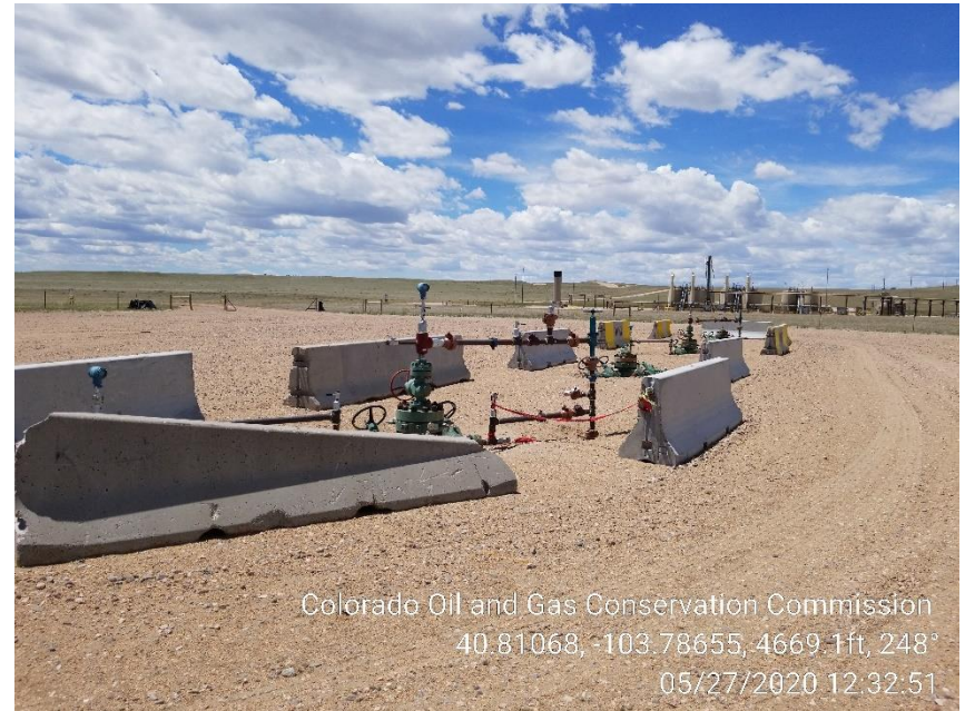
Photo 2 – Wellheads – Signs missing
