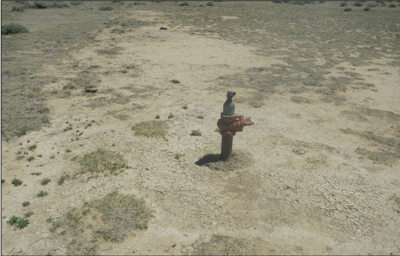
Photo 2. There is a pipe riser that remains at the tank battery location north of the well site at Lat/Long:38.42173,-103.01423.
