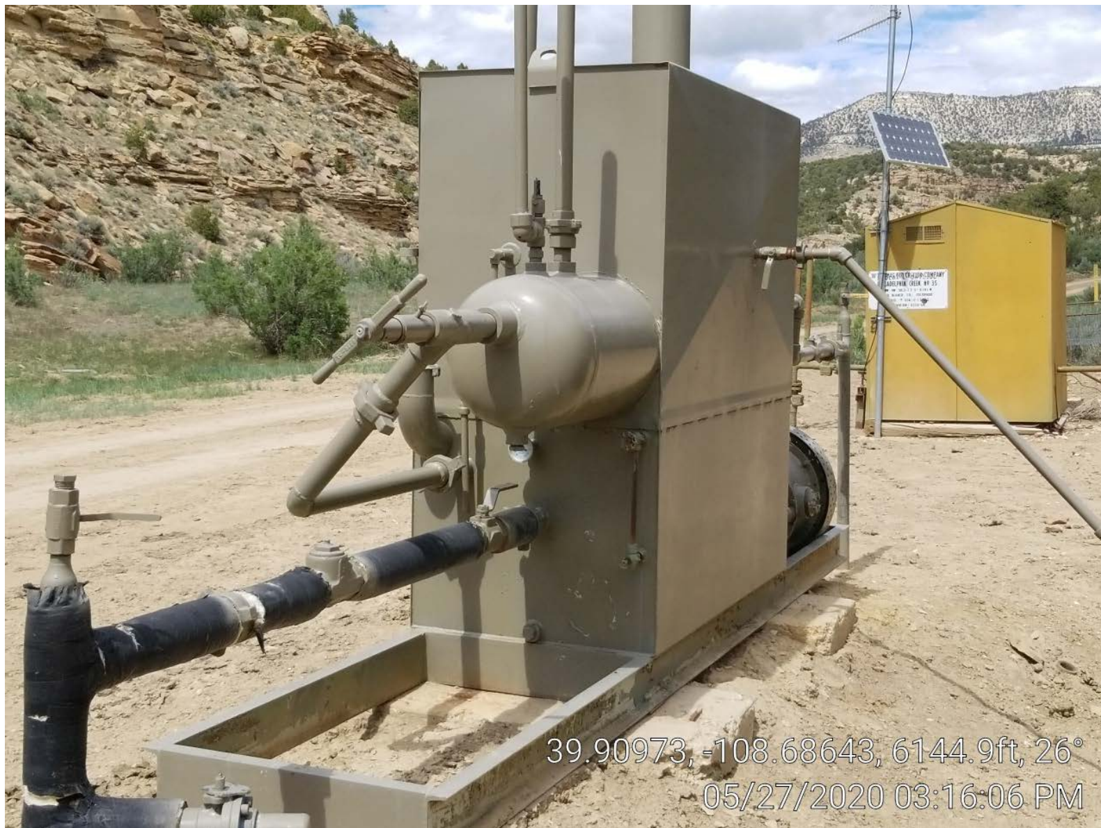
Photo 2. Separator & meter building.
