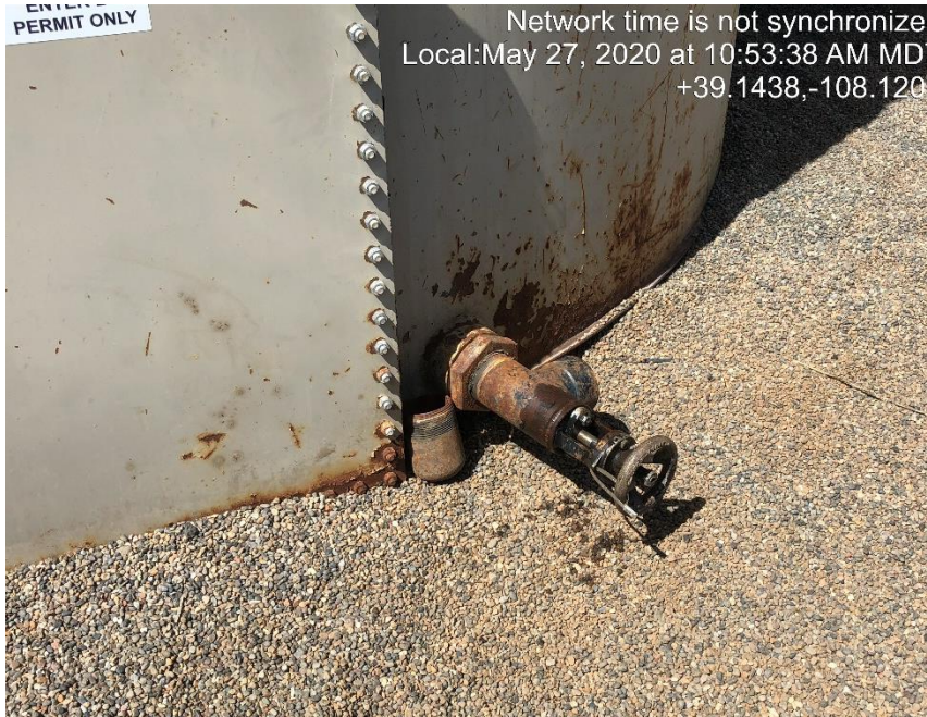
Photo #1261 Multiple unused bull plugs in tank containment.
