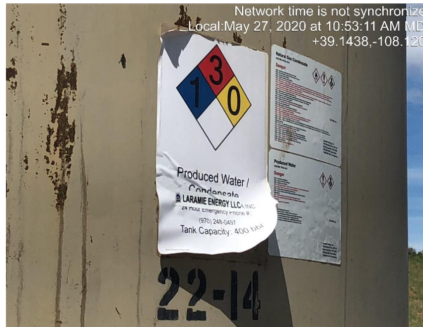
Photo # 1260 Tank label peeling off tank and tank capacity is inaccurate.
