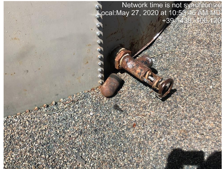
Photo #1262 Multiple unused bull plugs in tank containment.
