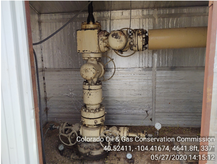
Photo #1 NGL C7A (05-123-32207) Injection Well Active Injection
