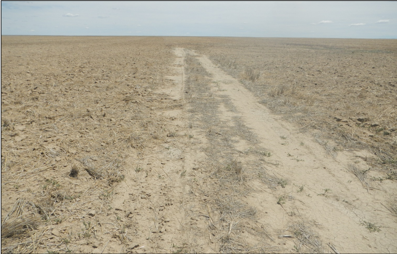
Photo 2. Facing east toward the access road which travels through the cropland. The former road has not been properly decompacted by ripping to 18 inches.
