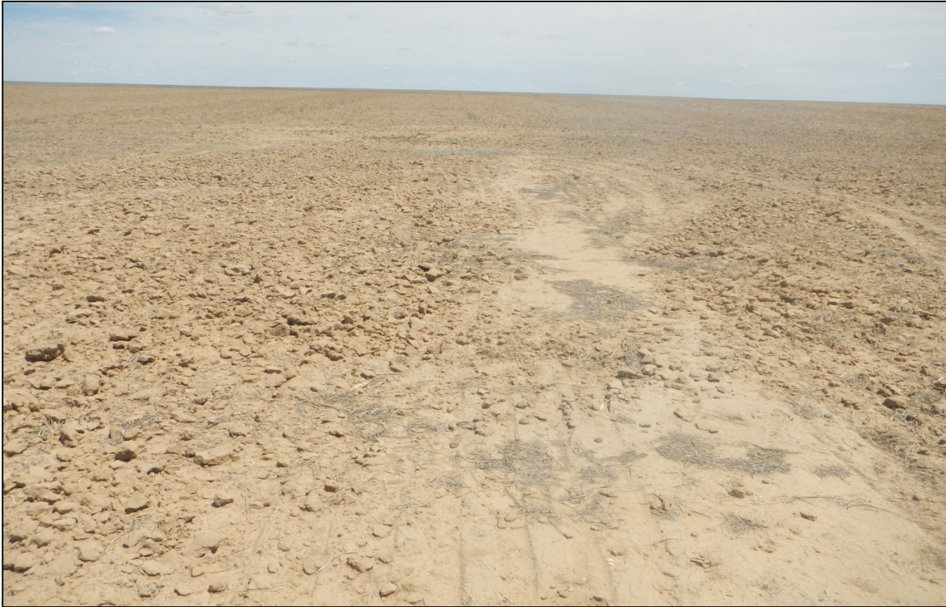
Photo 5. Facing east toward the location. All equipment has been removed from the location. The soils at the location are compacted and must be cross ripped to a depth of 18 inches.
