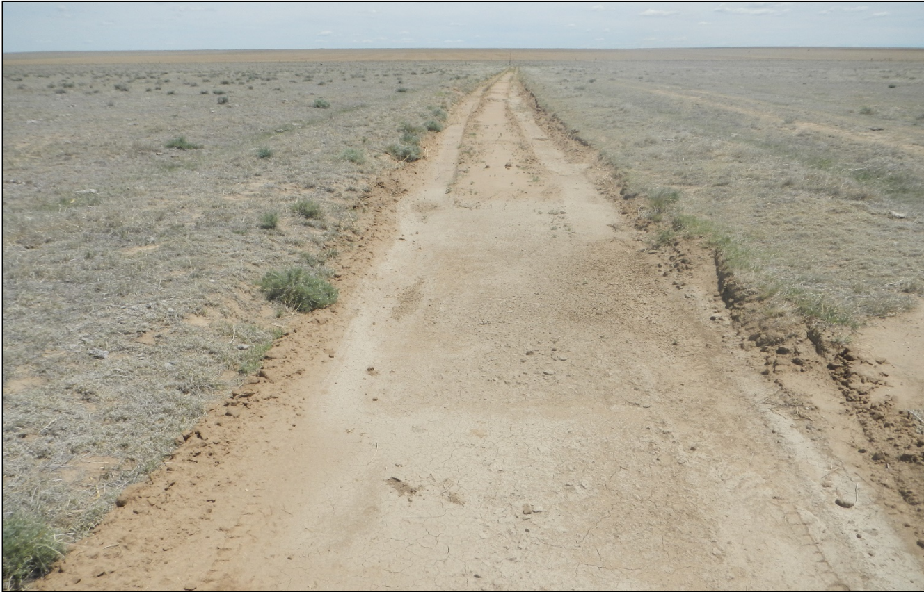
Photo 1. Facing east along the road used to access the well site. This road is rutting and degraded and needs to be repaired.
