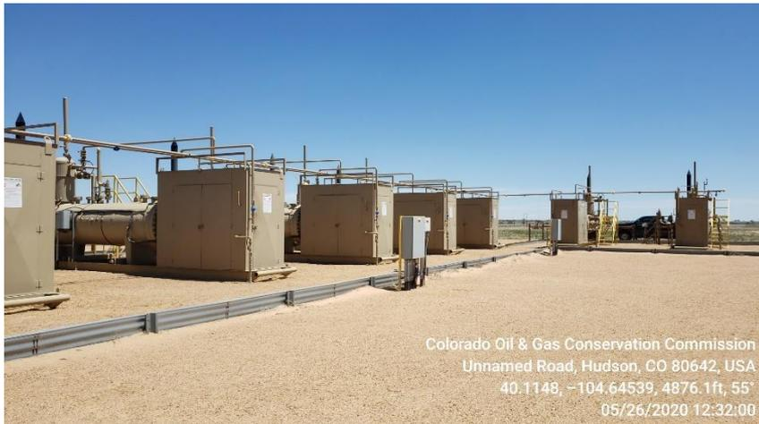
Photo 7 Horizontal Heated Separator
