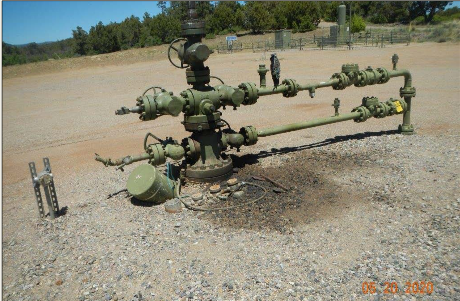
Photo 4. View of stained soils around the wellhead.
