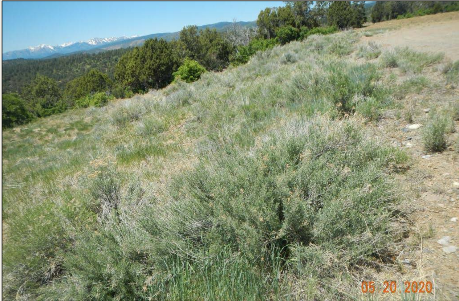
Photo 2. View of the western fill slope from the southwestern corner facing northward. Revegetation is progressing on the slope with grasses such as western wheatgrass and smooth brome, as well as shrubs such as rubber rabbitbrush.
