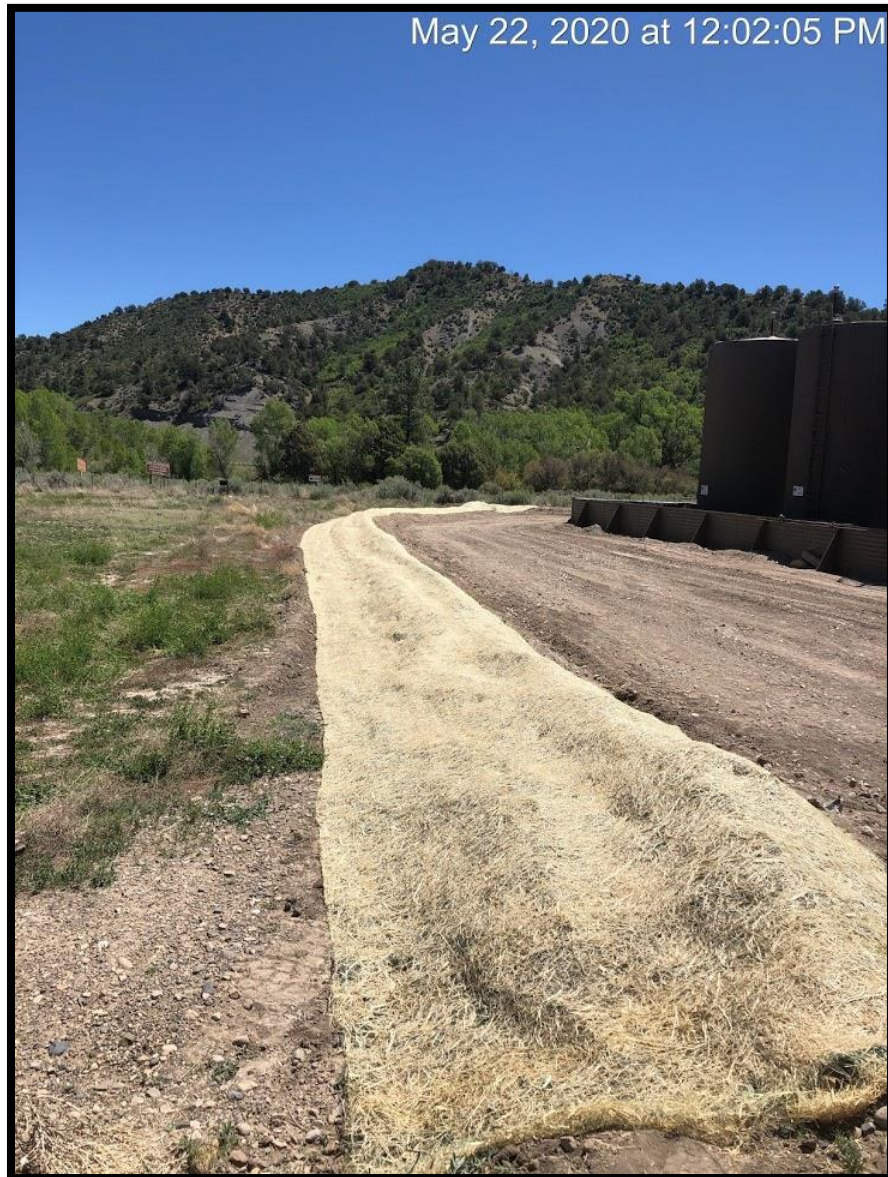
Eastern Half of North Berm and North portion of East Berm was recontoured, seeded and erosion blankets were placed on 5/22/20
