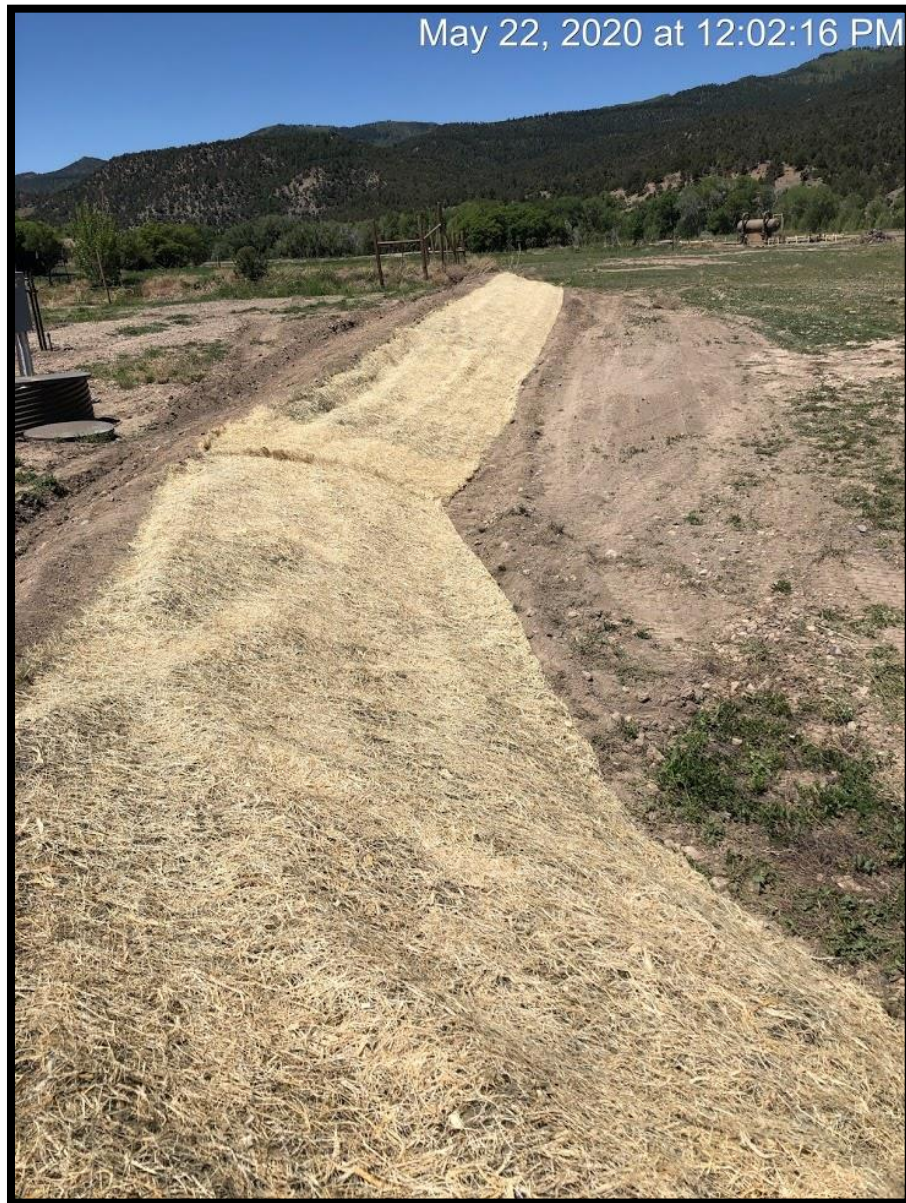
Western Half of North Berm was recontoured, seeded and erosion blankets were placed on 5/22/20
