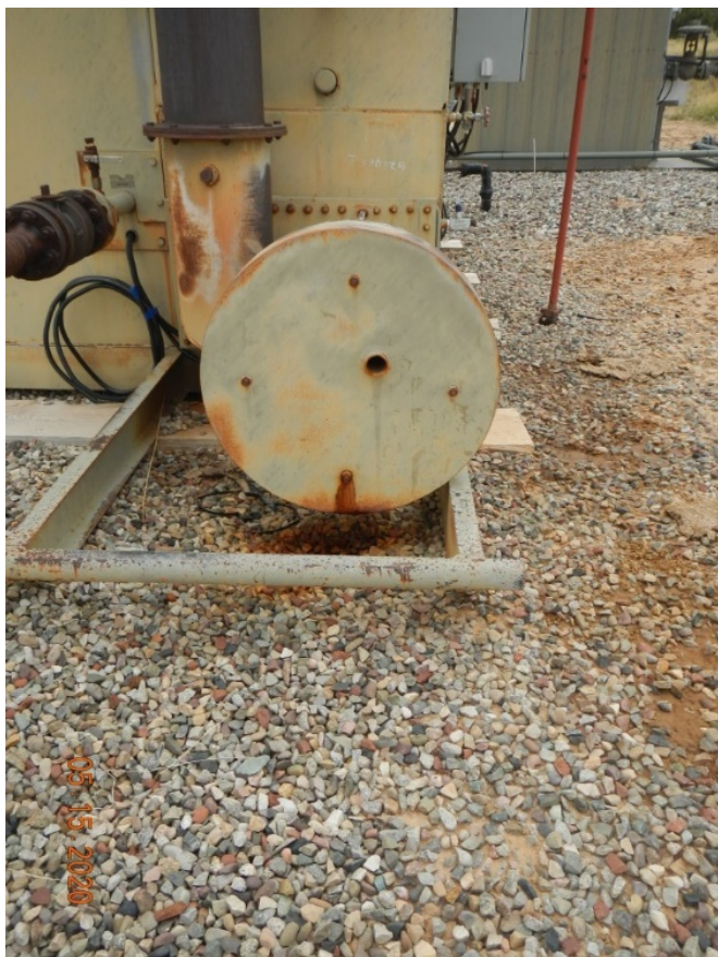
Photo#5: Staining at back of separator
