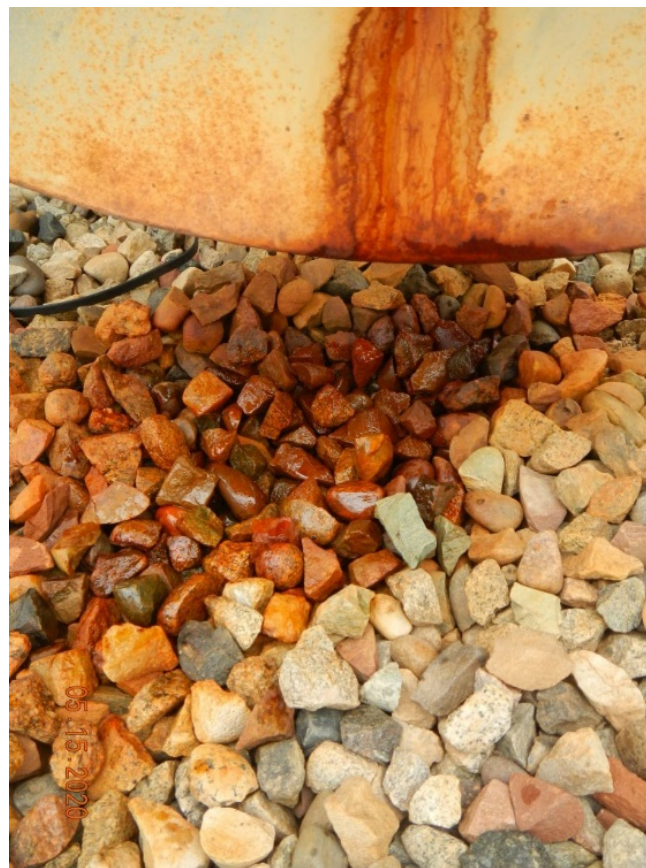
Photo#6: Staining at back of separator.
