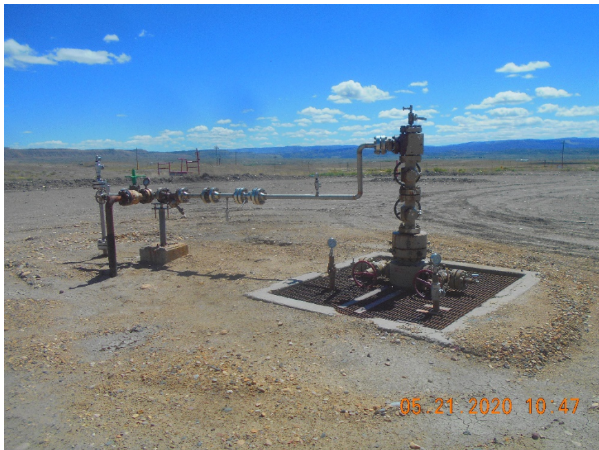
Injection wellhead
