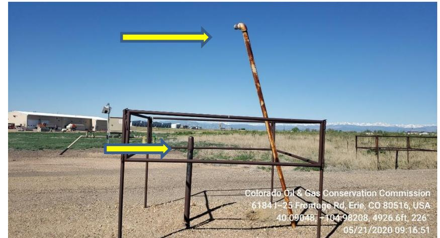
**Photo 7 unused unmarked no LOTO on Flow line riser**
