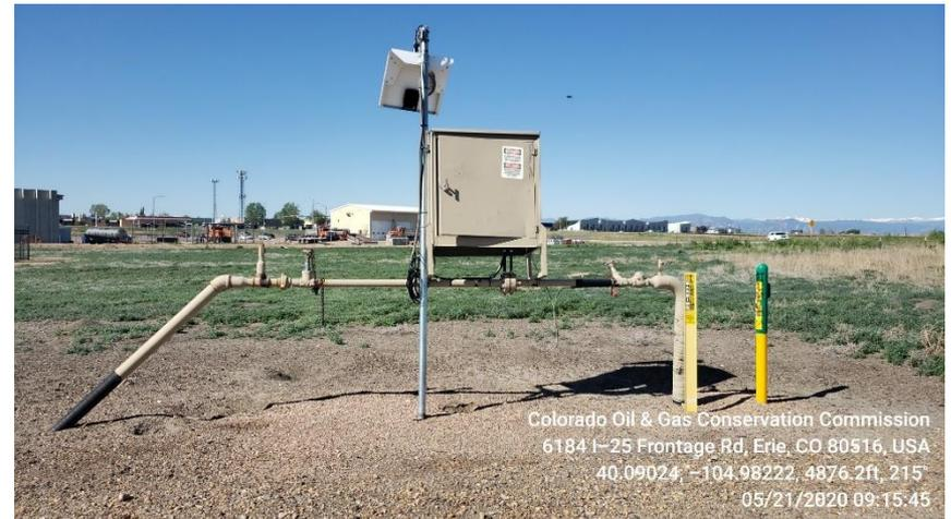
**Photo 5 ECD and Horizontal Heated Separator**
