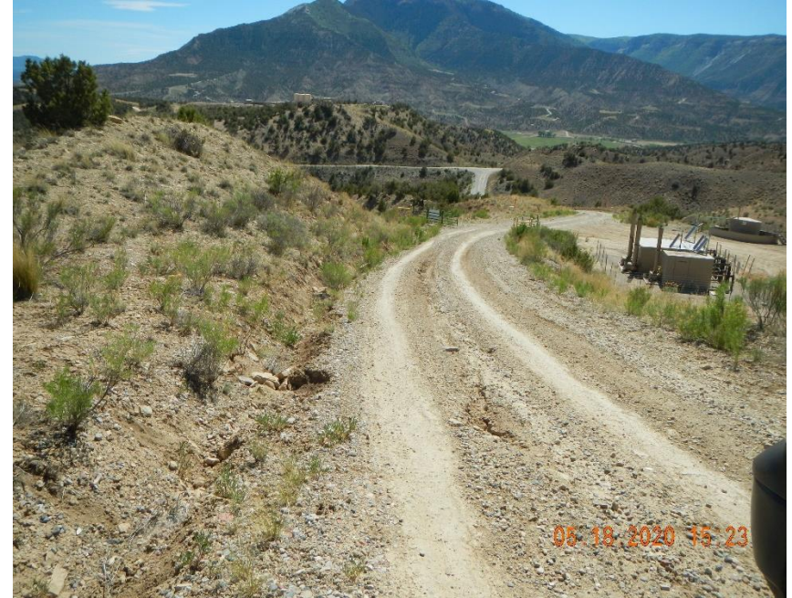
Storm water damage on access road to location.
