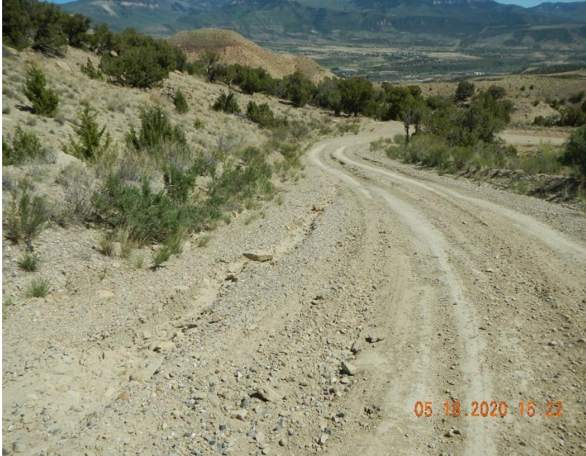
Storm water damage on access road to location.
