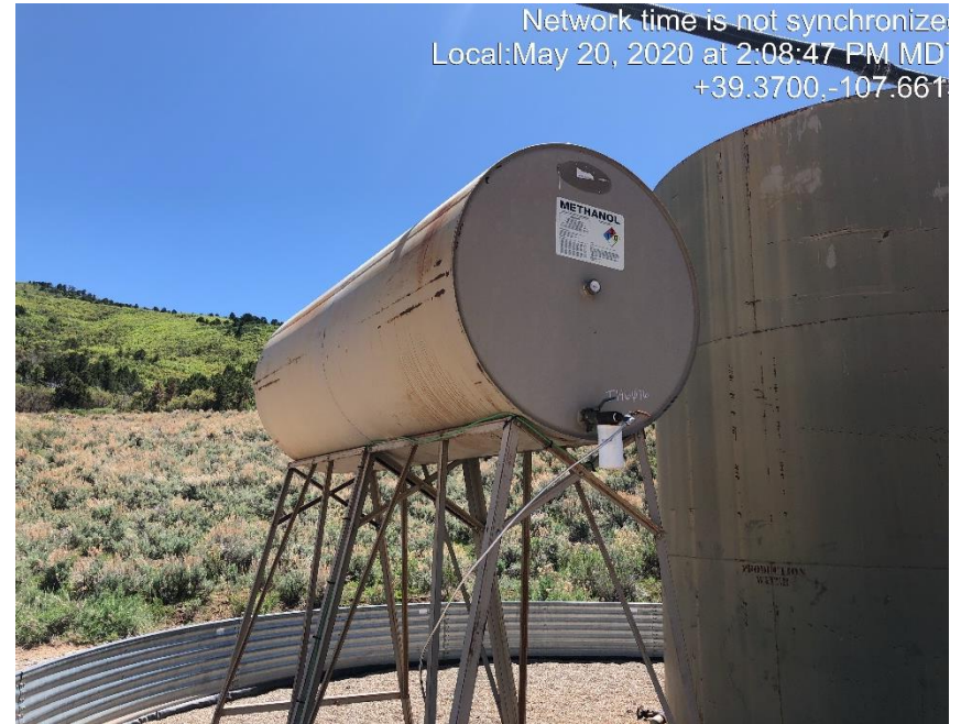
Photo #1230 Methanol tank not properly labeled.
