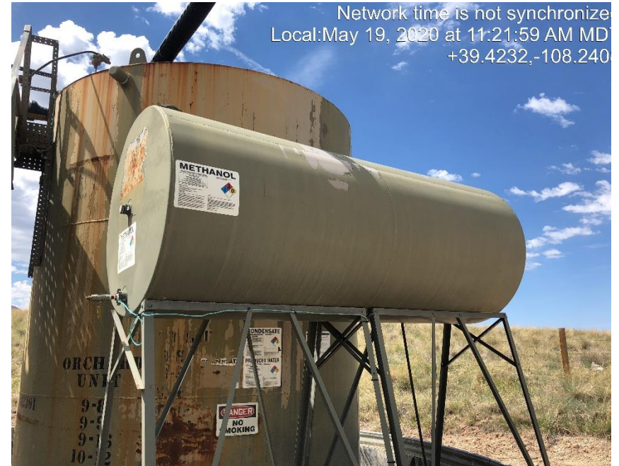
Photo #1210 Methanol tank not properly labeled.
