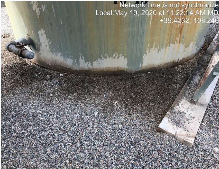
Photo #1211 Stained gravel in tank containment.
