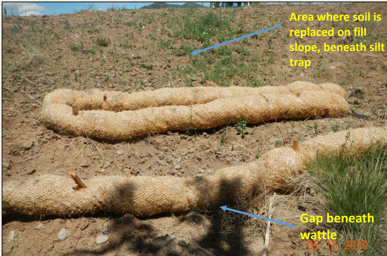
Photo 3. View of area on southern fill slope where sediment trap was breeched and is repaired. Area is replaced with soil, and appears to have been seeded. Wattles in place as secondary containment are not installed properly as they are not trenched into soil.
