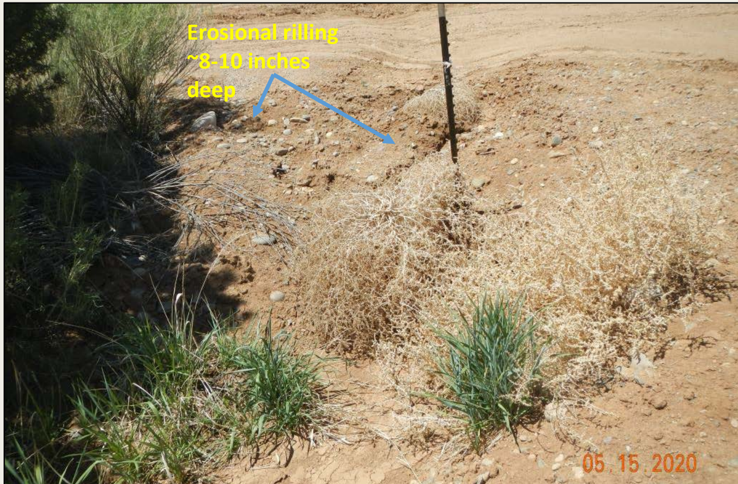
Photo 4. View of area where erosion is occurring where culvert crosses the access road near the well pad entrance. Additional stabilization is needed here.
