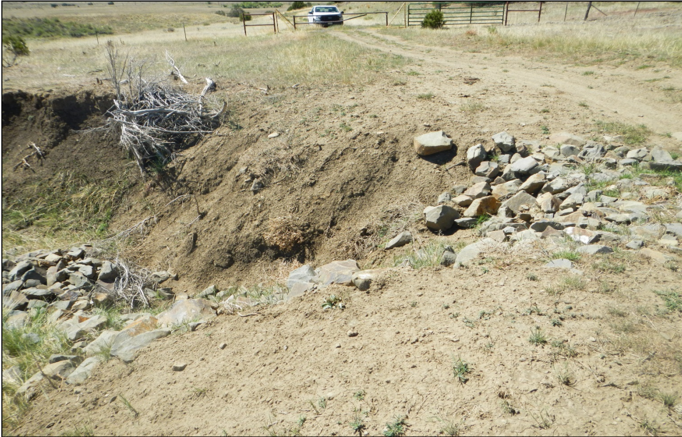
Photo 5. Facing back toward the south near the cattleguard. The road crossing near the drainage will require BMP maintenance. The rock rip rap has been washed out in this area.
