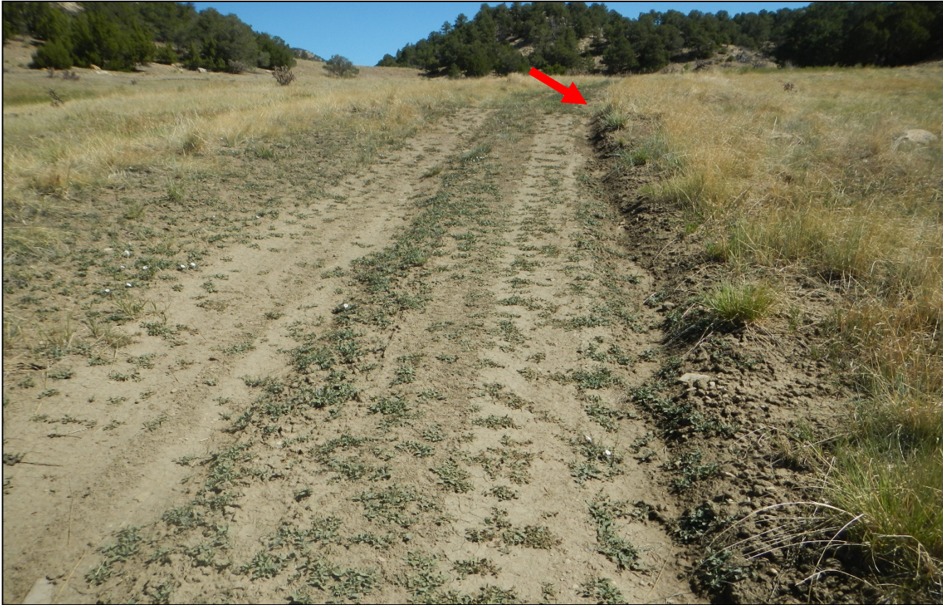
Photo 2. Facing north along the access road. There is an erosion channel that has developed overtopping water bar shown at red arrow.
