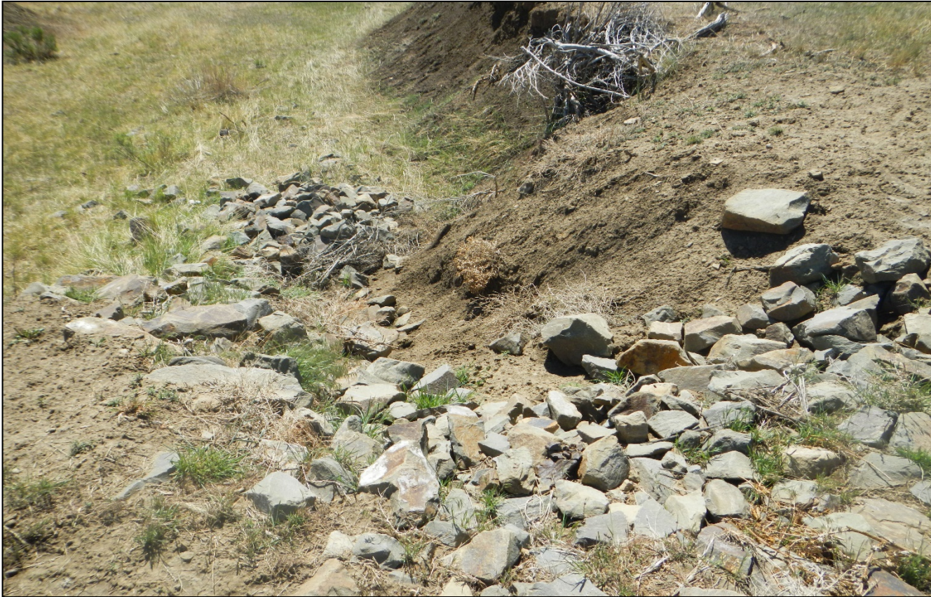
Photo 6. View of rock rip/rap that has been displaced will need to be repaired.
