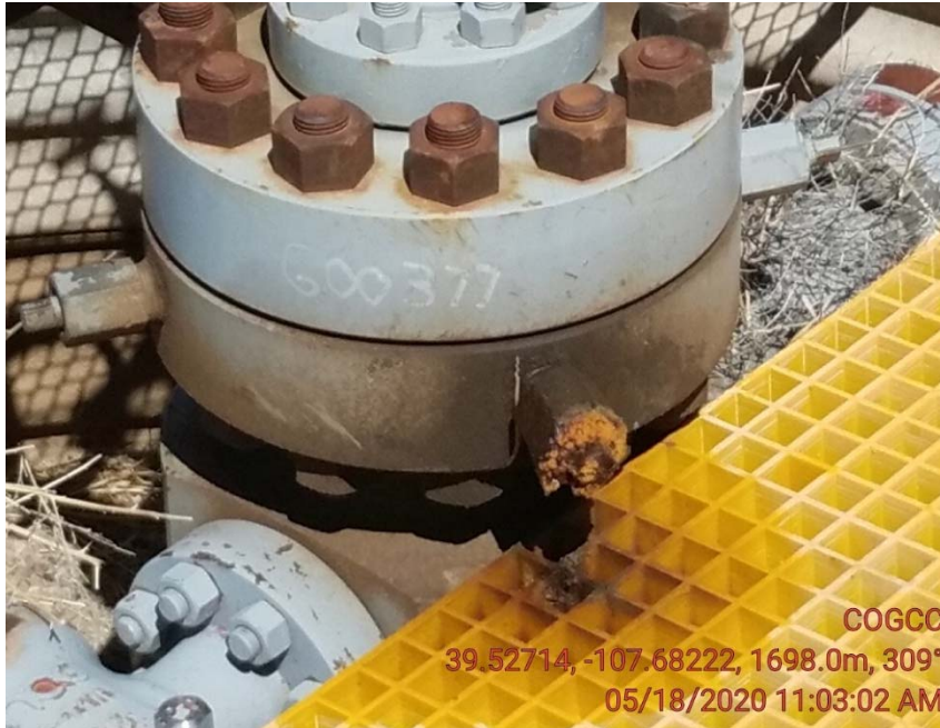
Dog nut is leaking
