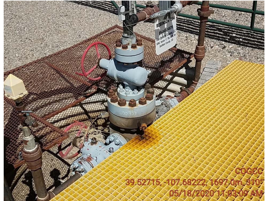
Dog nut is leaking
