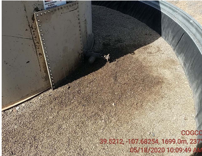
Staining under and around tank valve
