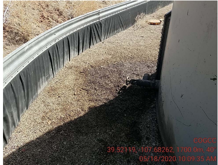
Staining under and around tank valve
