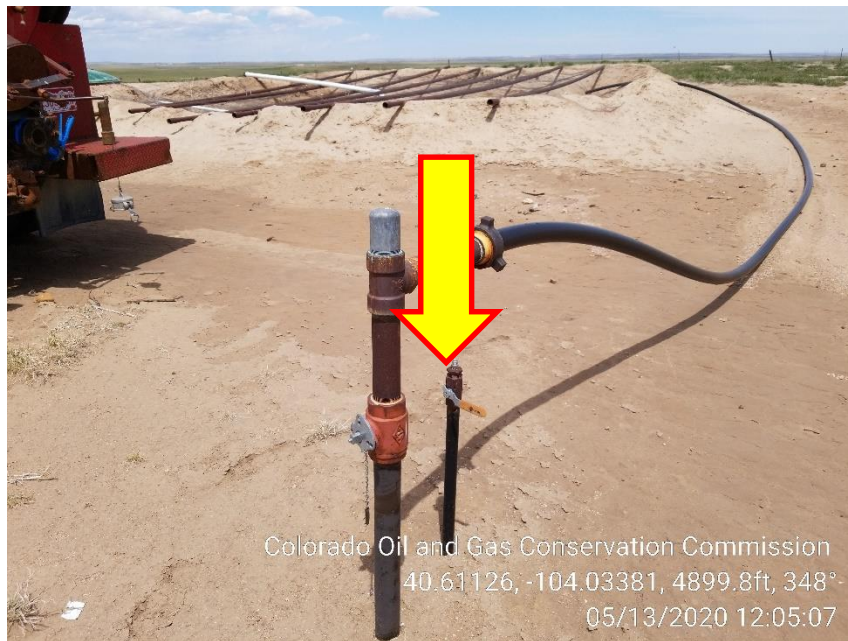
Photo 5 – Unmarked 1" Riser SE of Pit
