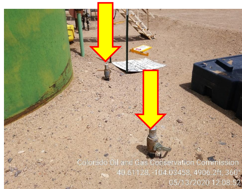
Photo 6 – Unmarked 2" Risers SE of Crude Oil Tanks
