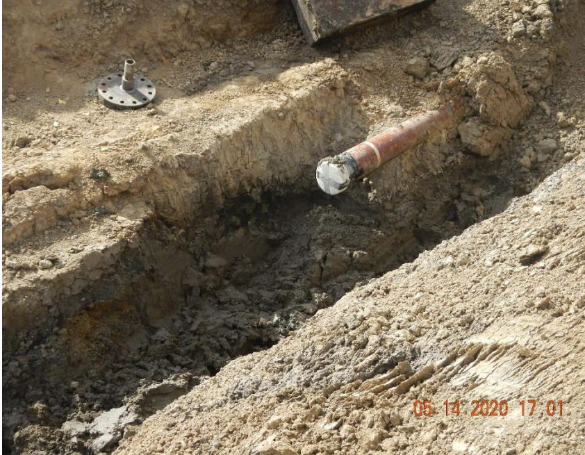
Fiberglass pipeline where water was being purged from.
