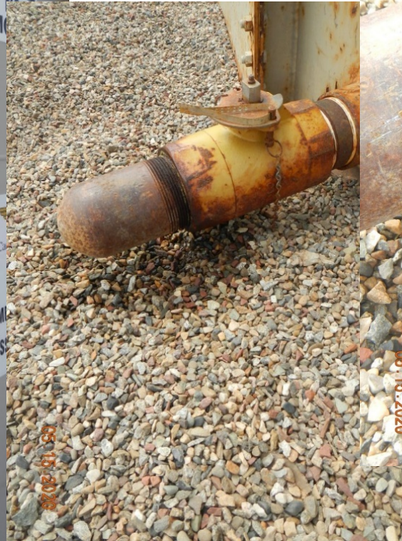
Photo#3: Drip at valve, Tank 1.
