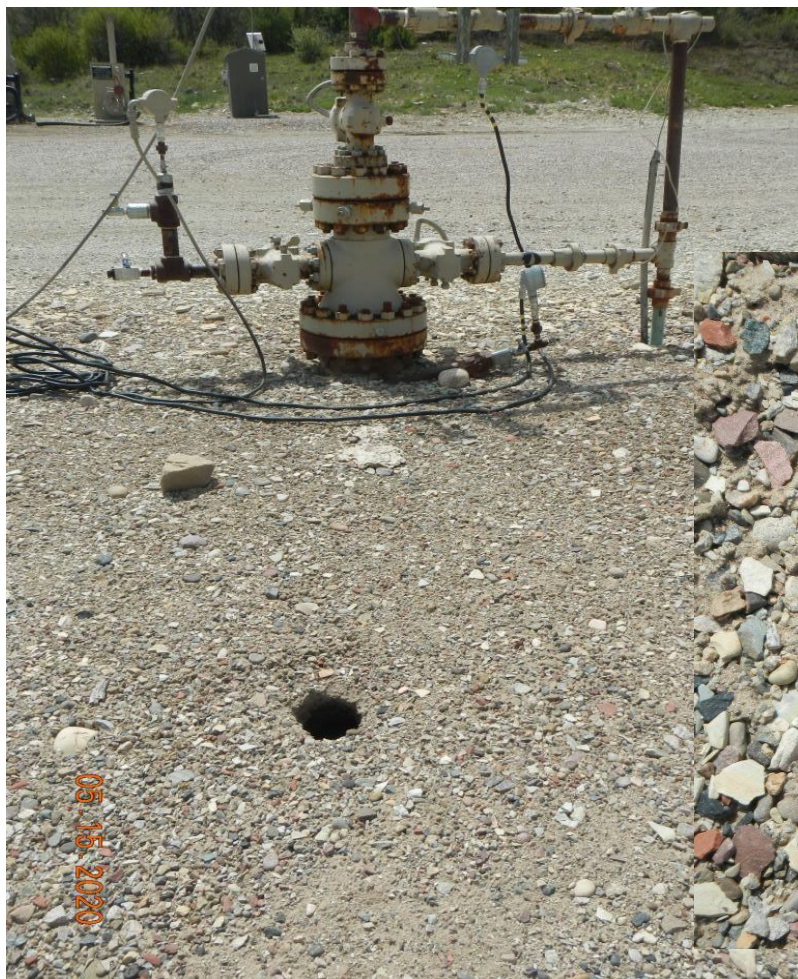
Photo#4: Subsidence NW of Rose Ranch Wellhead.
