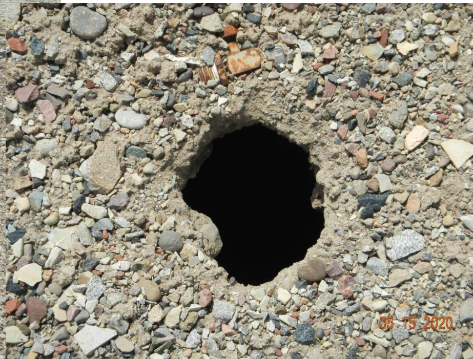
Photo#5: Subsidence NW of Rose Ranch Wellhead.
