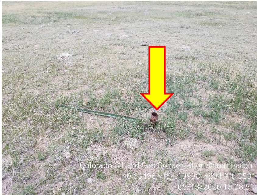
Photo 3 – Unmarked Deadman Anchor
