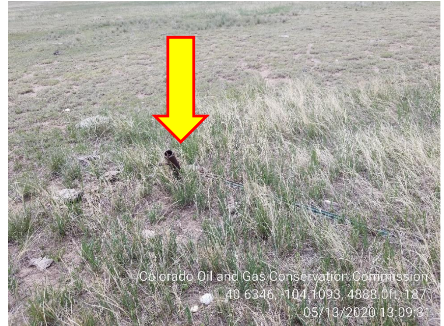
Photo 4 – Unmarked Deadman Anchor
