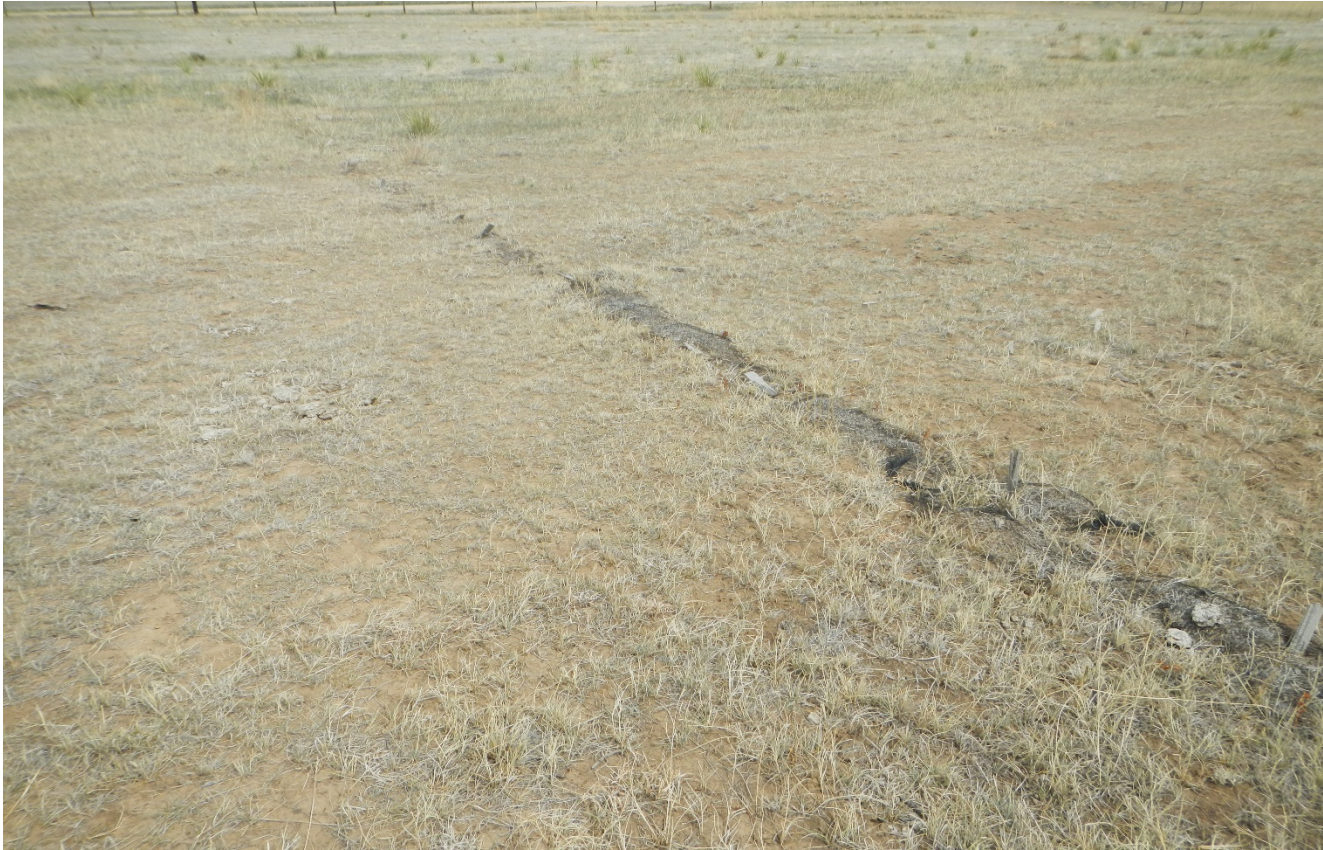
Photo 5. The degraded wattles remain at the location. The plastic netting and stakes need to be removed.
