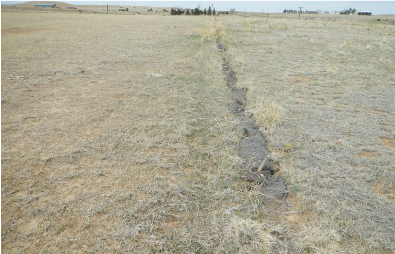
Photo 6. The degraded wattles remain at the location. The plastic netting and stakes need to be removed.
