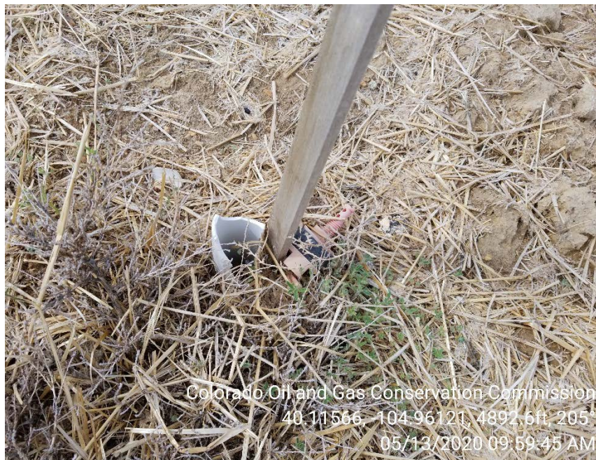
Photo 3 – Monitoring well; damaged and uncapped
