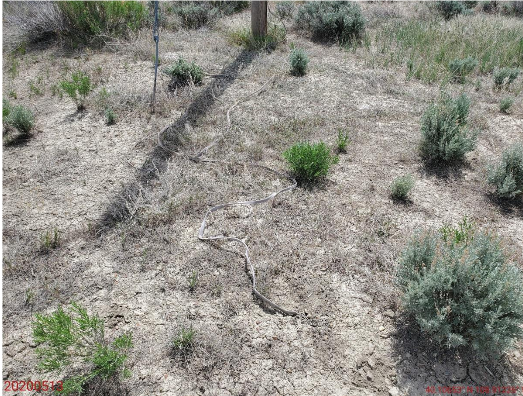
Photo 3: Photo shows exposed wire that had cut at the utility pole.
