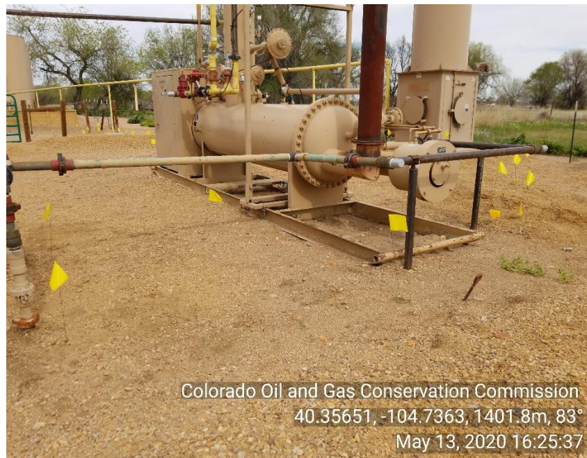
Photo 5: Separator not anchored
