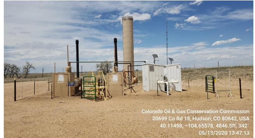
**Photo 6 Horiz. Heated Sep., ECD and gas meter runs**
