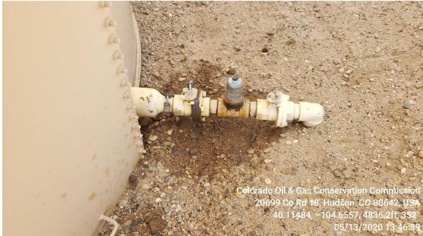
**Photo 5 stained soil under valve on crude oil tank**
