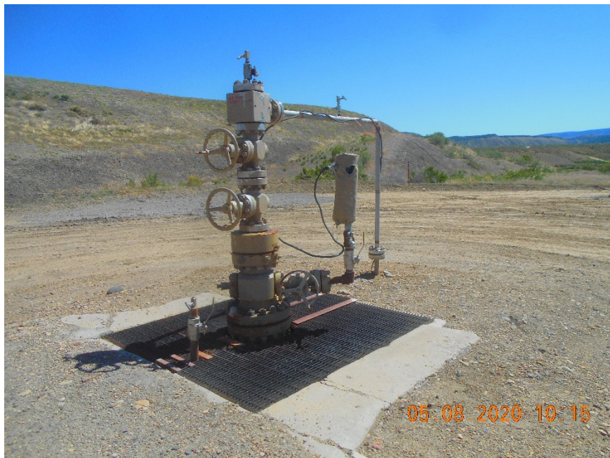
Injection wellhead
