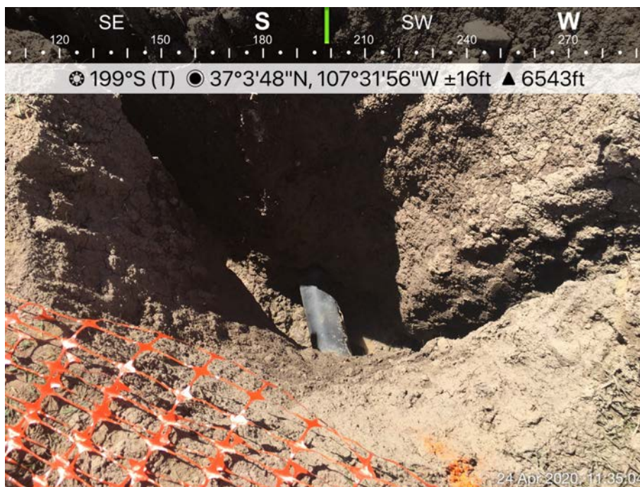
Photo 14: Excavation of ruptured pipeline, 4/24/2020.
