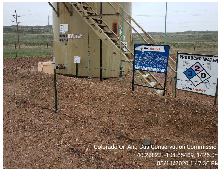
Crude oil tank earth berm
