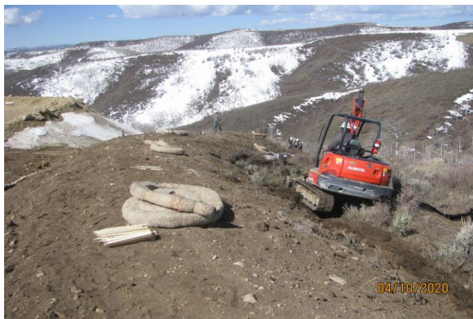
Wattle Installation on the C.C. 610-21-41 Pad
