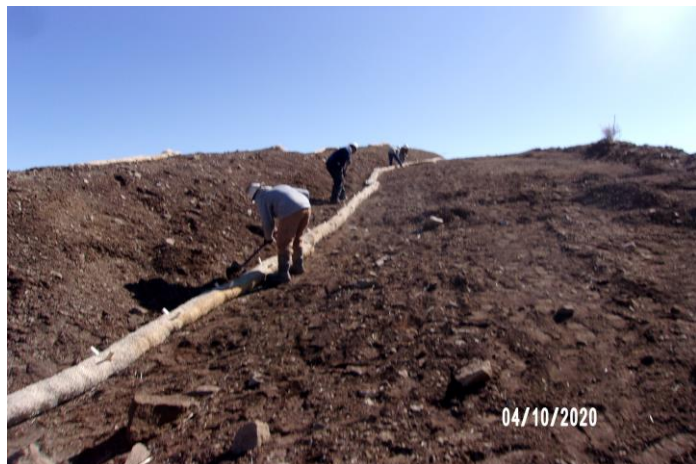
Wattle Installation on the C.C. 610-21-41 Pad
