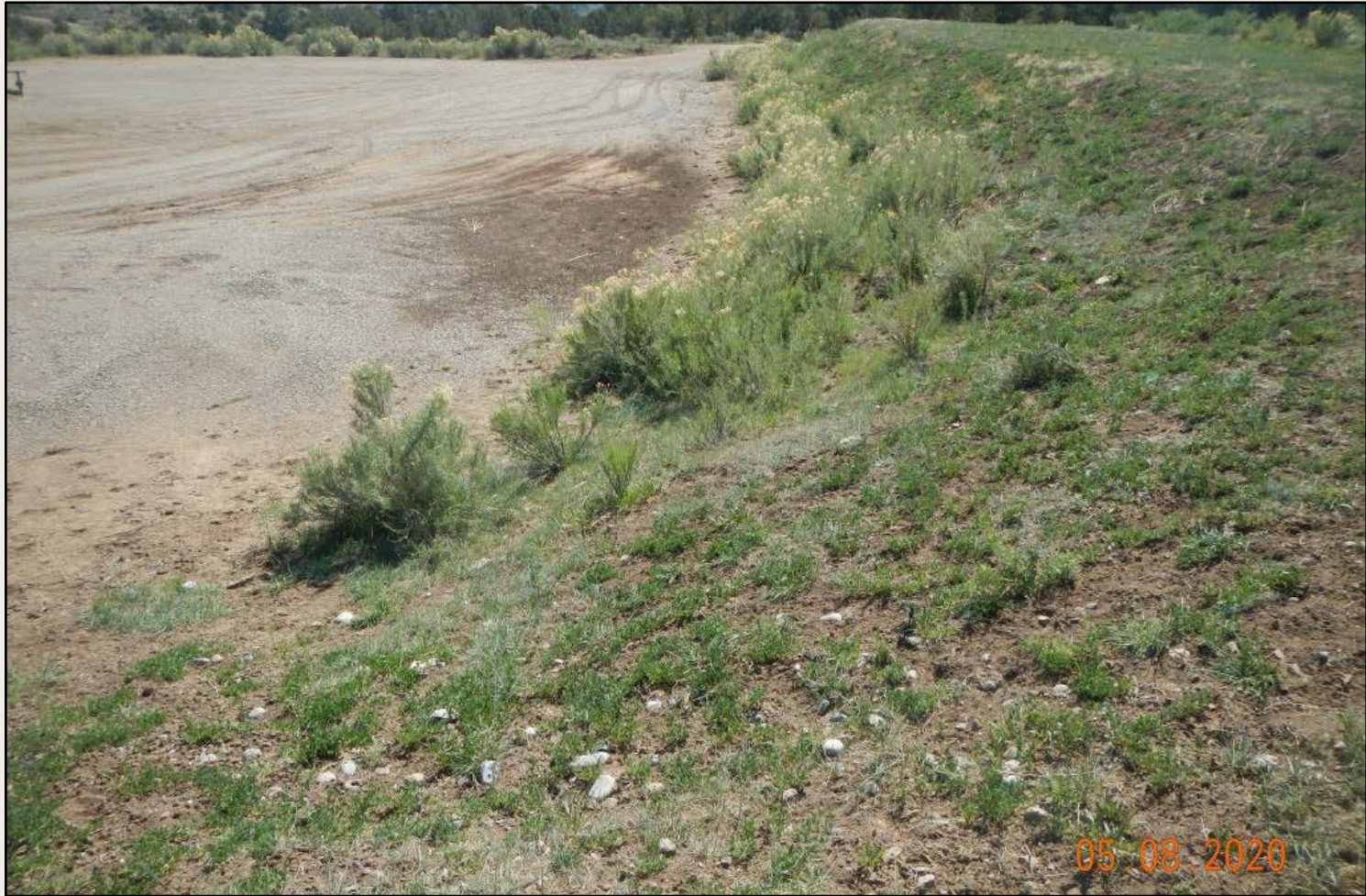
Photo 3. View of the central fill slope from the southwestern corner facing eastward. Revegetation is progressing with rubber rabbitbrush and grasses such as western wheatgrass.
