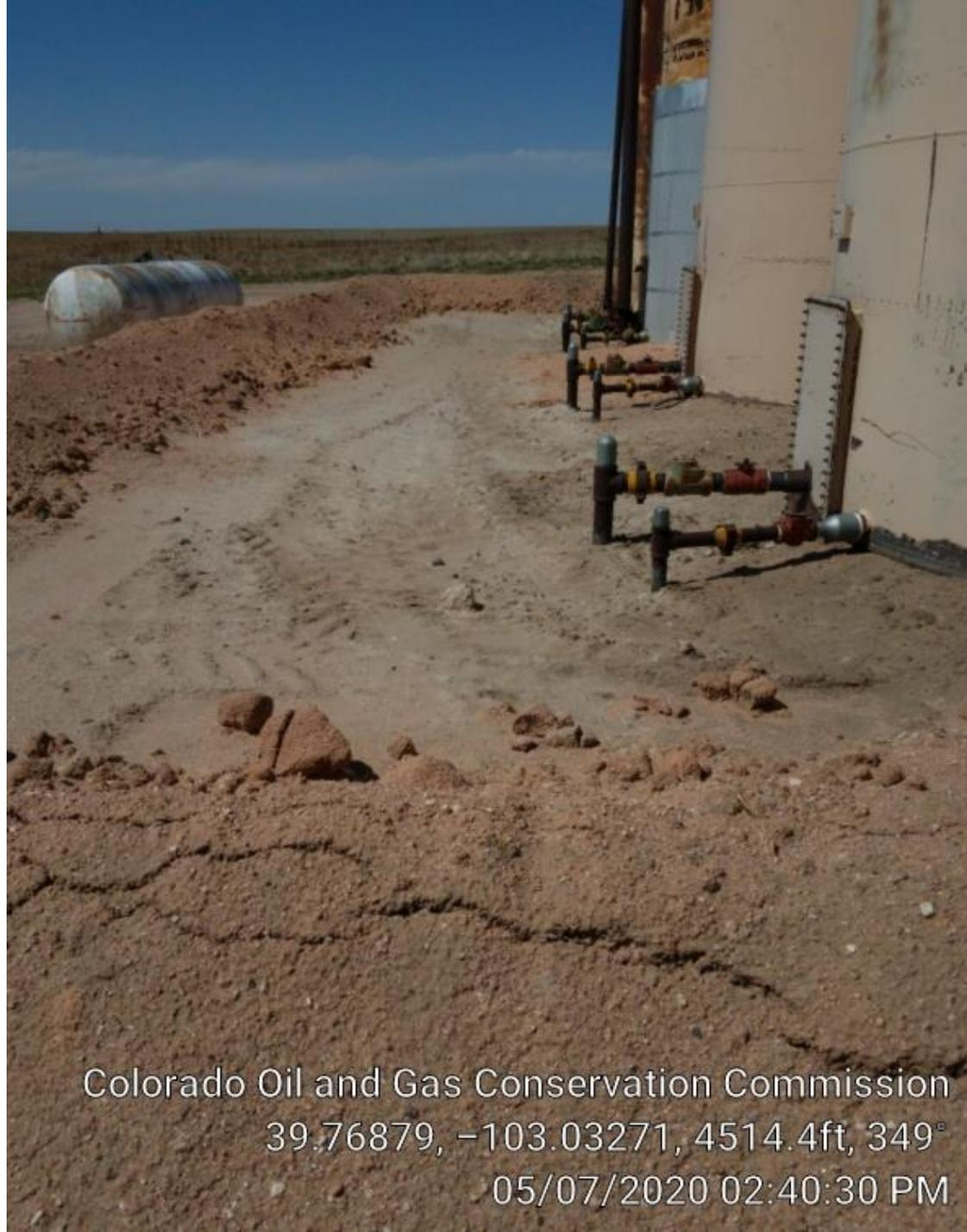
Absorbent natural clay material put at base of berms after spill in berms.
