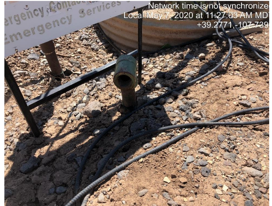
Photo #1140 Flow line riser not LO/TO.
