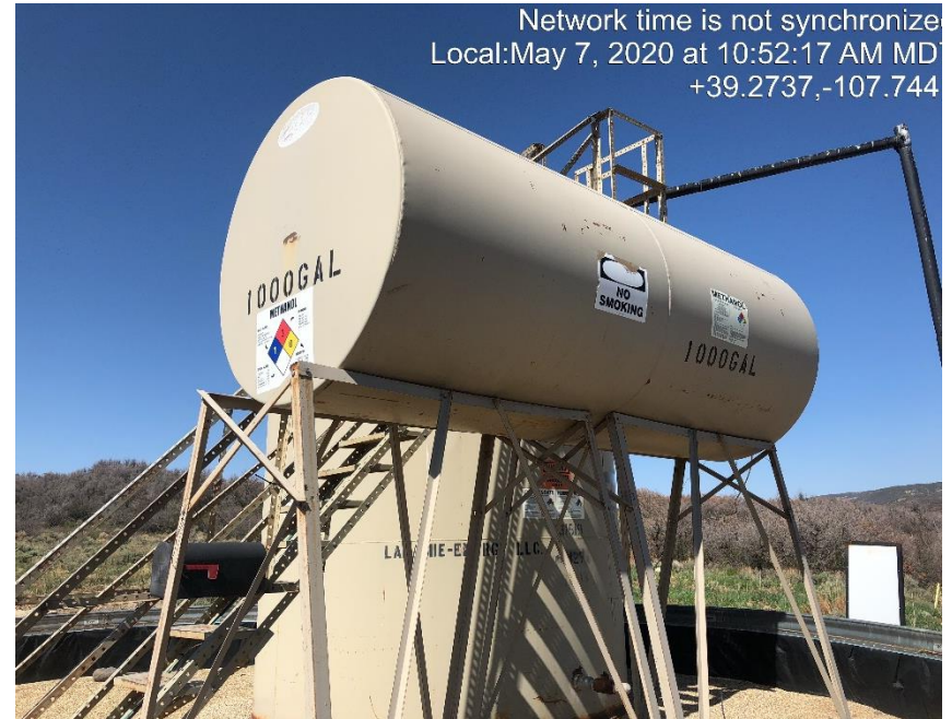
Photo #1138 1000 gallon tank not properly labeled.
