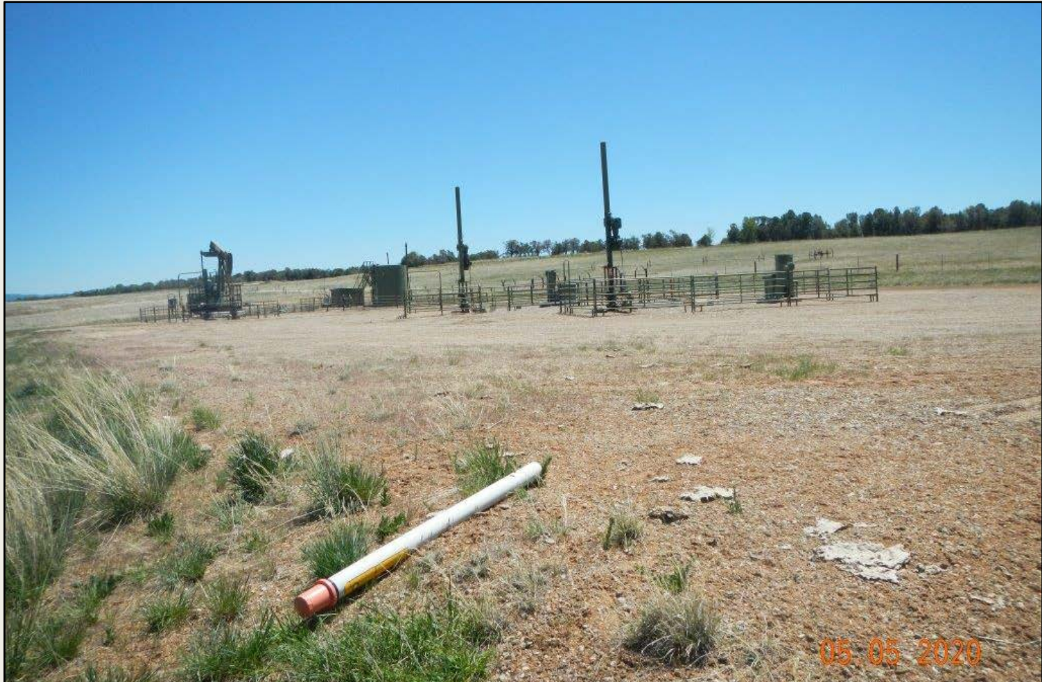
Photo 1. View of the project area from the northwestern corner facing center. Electrical cover is knocked down and needs to be repaired.
