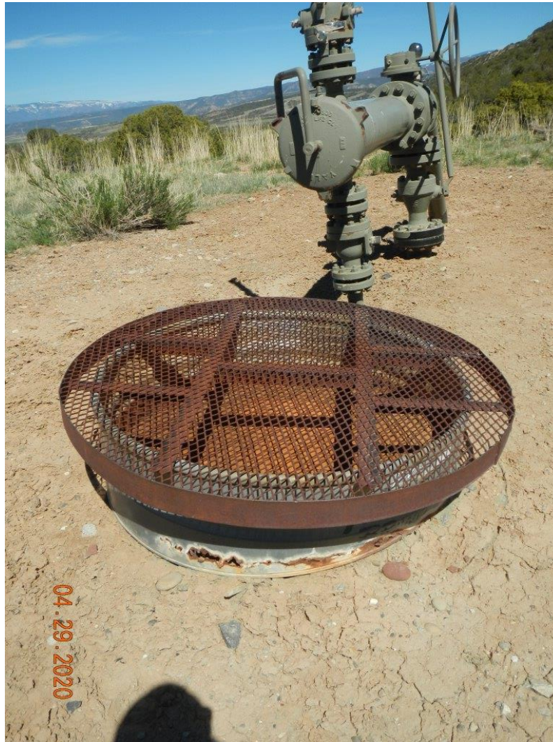
Photo#2: Tank with holes at base.
