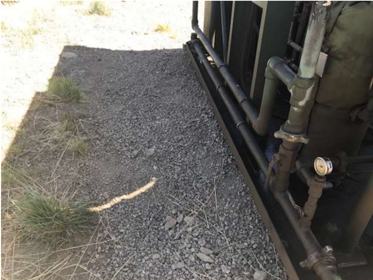
PHOTO 5: THE IMPACTED SOIL/GRAVEL NEAR THE LIQUID RING COMPRESSOR WAS REMOVED FROM THE LOCATION.
