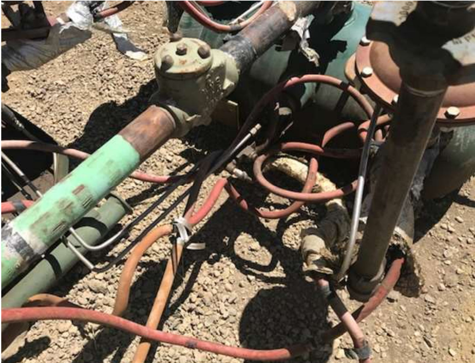
PHOTO 4: THE IMPACTED SOIL/GRAVEL NEAR THE LIQUID RING COMPRESSOR WAS REMOVED FROM THE LOCATION.
