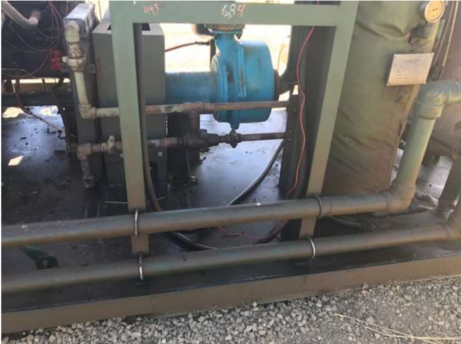
PHOTO 3: THE FLUID ACCUMULATION WAS REMOVED FROM THE CONTAINMENT OF THE LIQUID RING COMPRESSOR AND THE SKID WAS CLEANED
