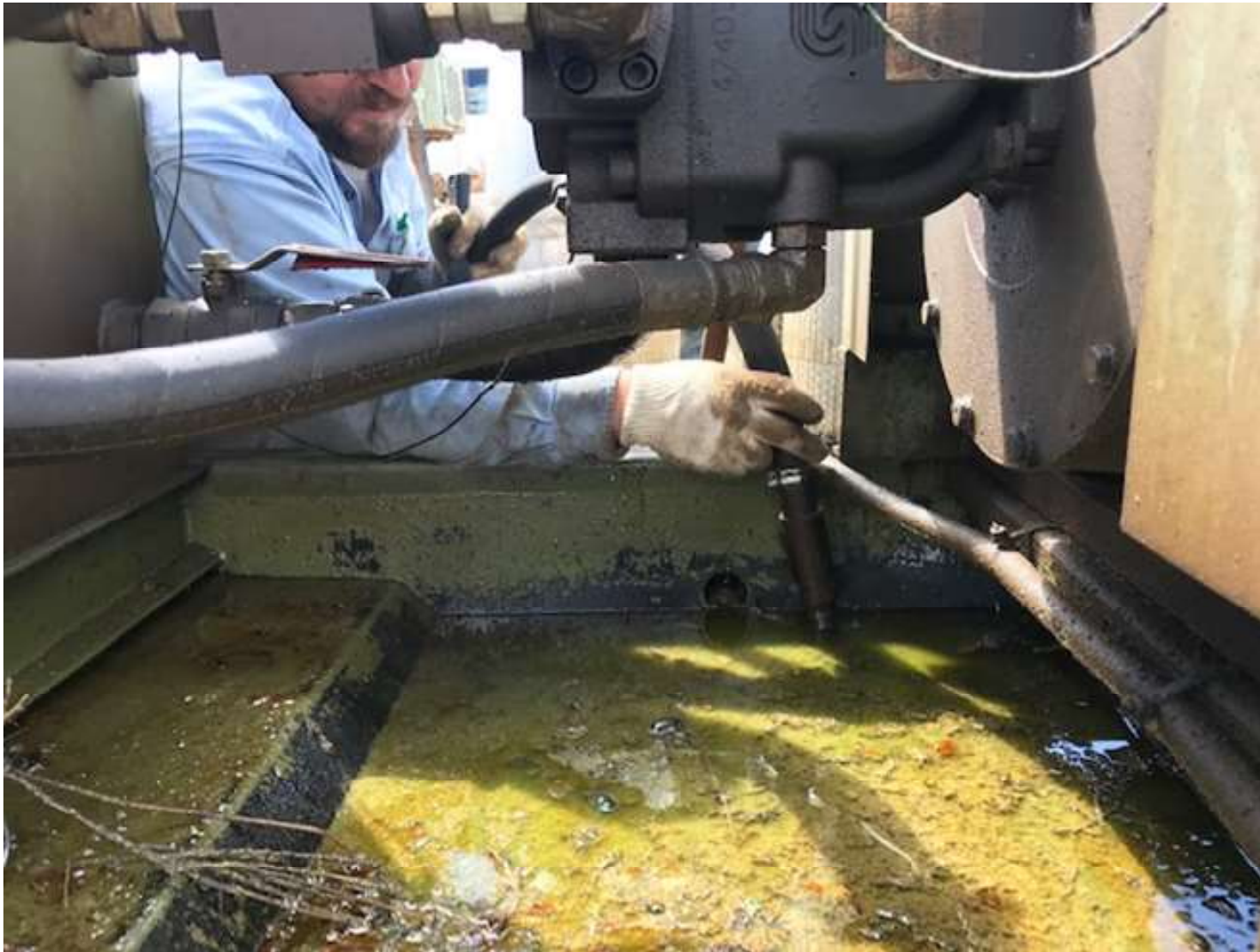
PHOTO 2: THE FLUID ACCUMULATION WAS REMOVED FROM THE CONTAINMENT BELOW THE ENGINE.
