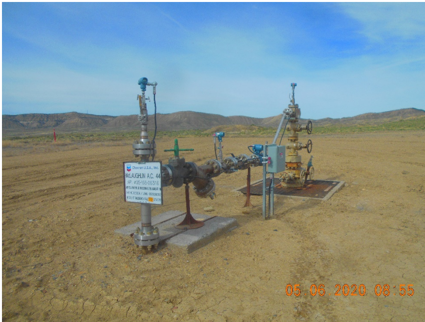
Injection wellhead
