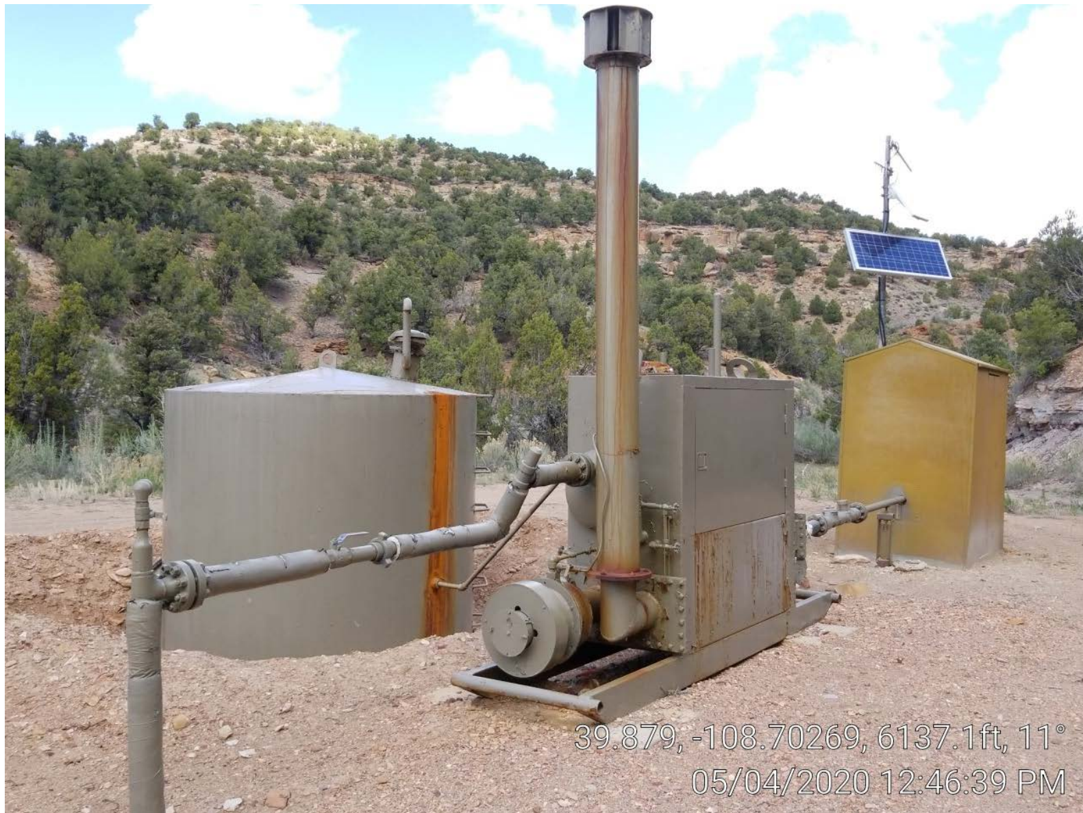
Photo 2. Tank, separator, and meter building.
